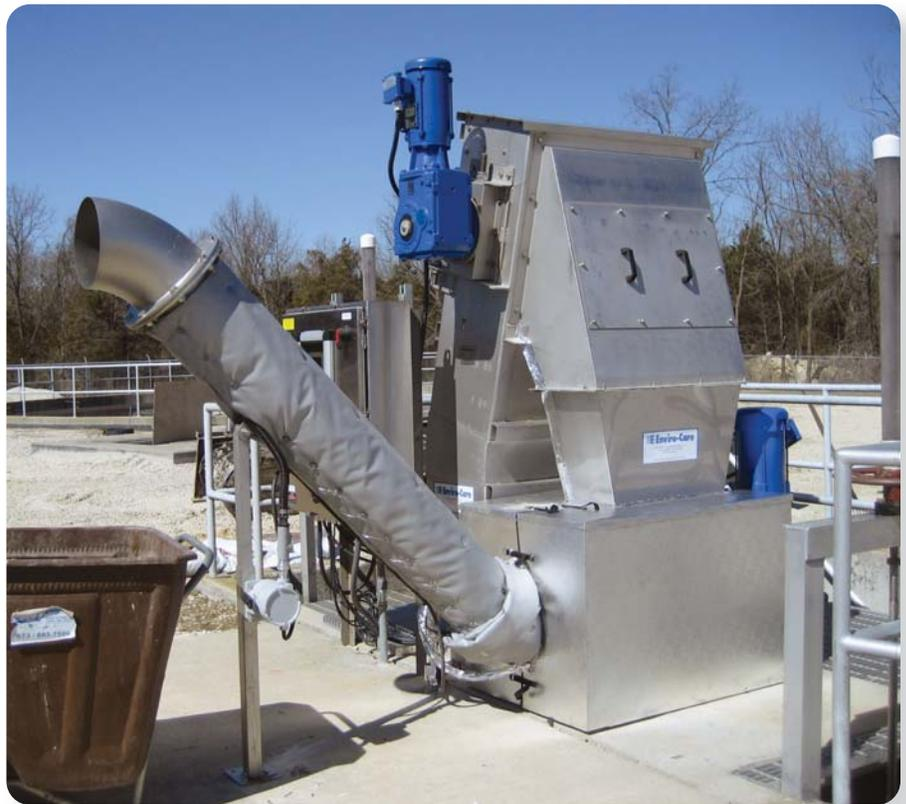
Flo-MultiRake screen and Flo-WashPress installed at the Cuba MO WWTP headworks
