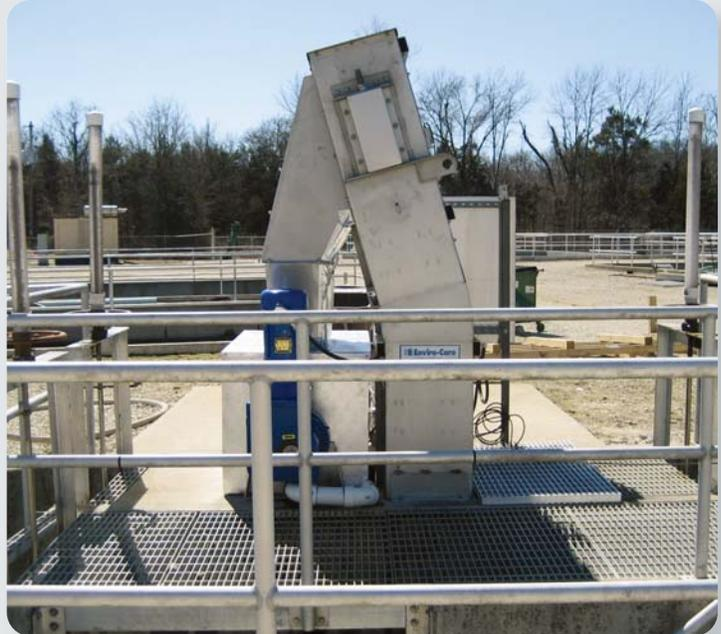
Flo-MultiRake Fine Bar Screen with 6 mm bar spacing installed at a 90° angle.
