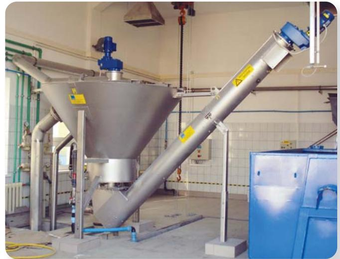
Flo-GritWash Unit Designed to Process 317 GPM of Grit Slurry
