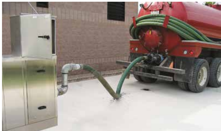
After the driver enters a hauler ID and the type of waste, a knife valve in the hauler station opens and the driver can begin discharging from the truck.
