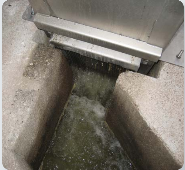
Multiple rakes reduce headloss.
