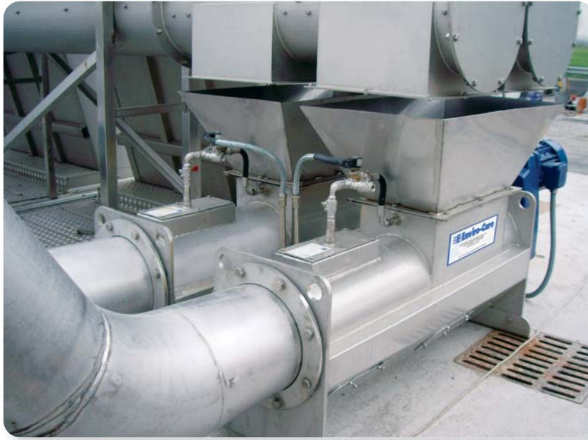
Two Flo-WashPress units receiving screenings from a conveyor system.
