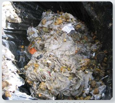
Screenings Removed by the Flo-MultiRake Fine Bar Screen
